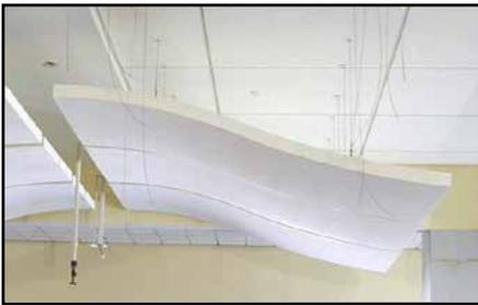
Four points are usually all that is necessary to suspend 2'x4' ceiling clouds in place. Six points are used for 4'x8' clouds. Keep corkscrews, hanger wires and anchors overtop in exact alignment, true and plumb.
