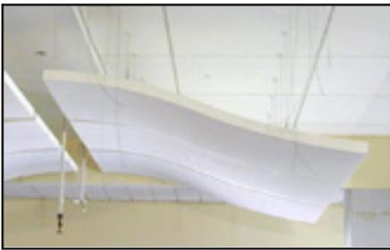
Four points are usually all that is necessary to suspend 2'x4' ceiling clouds in place. Six points may be used for 4'x8' clouds. Keep corkscrews, hanger wires and anchors ovetop in exact alignment, true and plumb.
