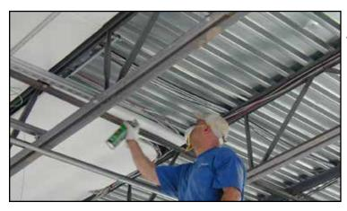
Underside of metal deck ribs are sprayed twice for best tack and secure bond.
