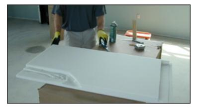
Shoulder and circular cut-outs made to suit panel conditions between open web joists. 2-inch thick panels can be back-cut extensively to fit over top bundled wiring and open web joist flange.
