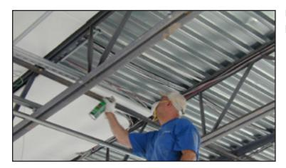
Underside of metal deck ribs are sprayed twice for best tack and secure bond.
