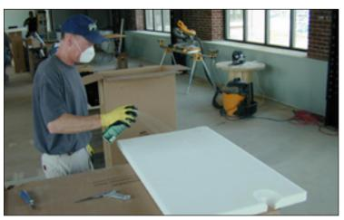
Once the panel has been properly fit to the deck, the back of the panel is totally spray coated using Hi Strength spray adhesive.
