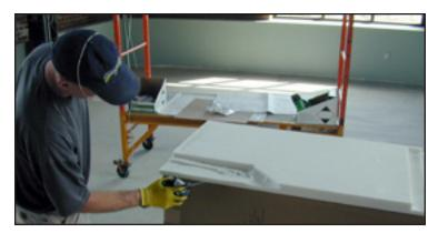
Apply spray adhesive to suit panel-to-panel, butt-edge conditions.
