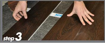
Engineered/Laminate wood floors, LVT/LVP are applied directly to Acousti-Top. Take care to avoid placing flooring seams directly in line with Acousti-Top seams.
