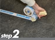
Tape seams of Acousti-Top with minimum 2" width tape
