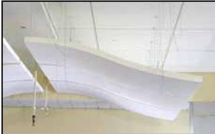
Four points are usually all that is necessary to suspend 2'x4' or 4'x4' ceiling clouds in place. Six points may be used for 4'x8' clouds. Keep corkscrews, hanger wires and anchors overtop in exact alignment, true and plumb.
