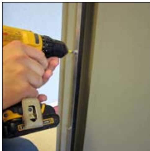
4. Install Jamb Seals to door frame.
