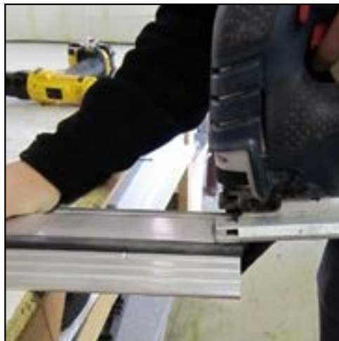
1. Measure & Cut for Threshold.
