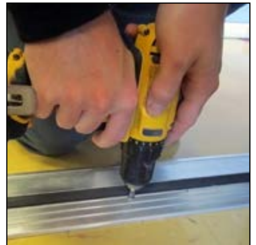
2. Install Threshold.
