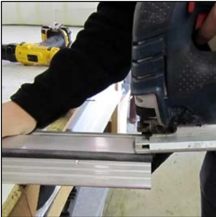
Measure, notch & Cut Threshold to required dimensions.
