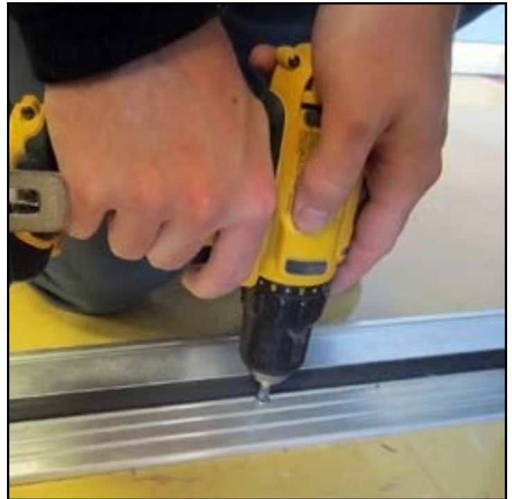
Install Threshold.
