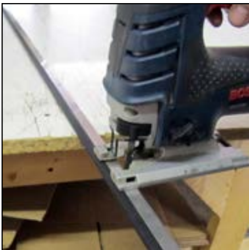
3. Measure & cut door jamb seals.
