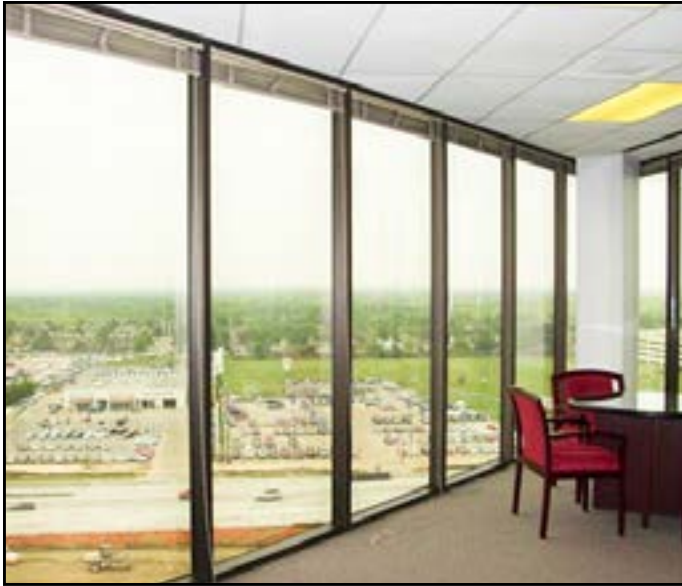
PrivacyShield ® Window Seal Kit applied over aluminum curtain wall construction for Balance America office suites, Houston, TX.
