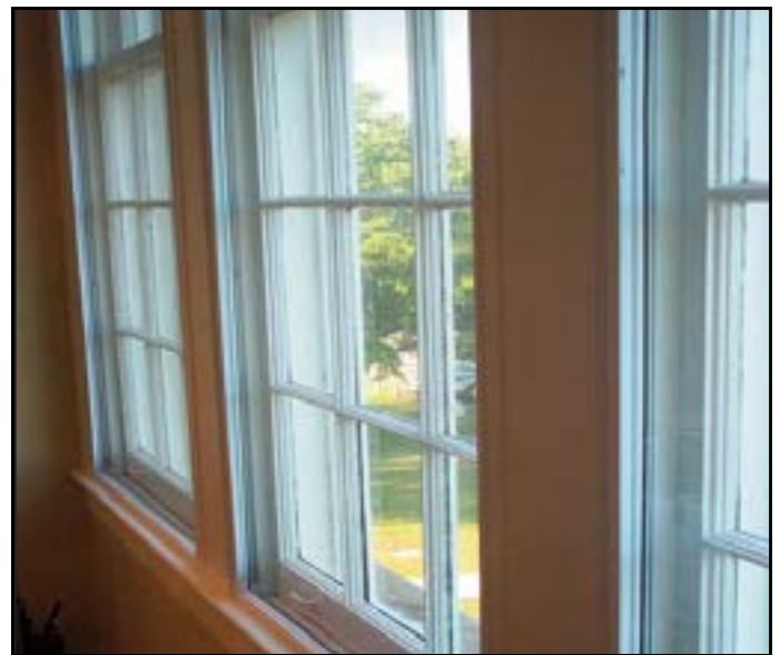
PrivacyShield ® Window Seal Kit applied over historic wooden windows at the Mary O'Keefe Cultural Center, Ocean Springs, MS.
